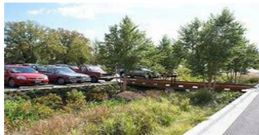
Parking lot Infiltration Island/planters
